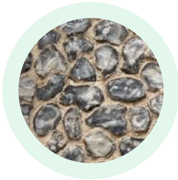
1. Flint Natural flint as locally sourced and a vernacular material found around Sussex
